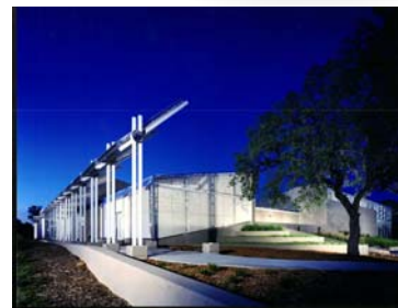
McConnell Foundation Maintenance Facility Redding, CA
