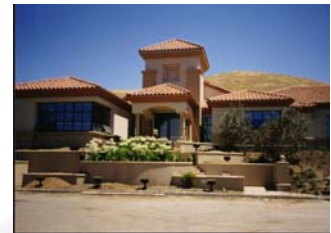
Mission San Jose Treatment Plant
