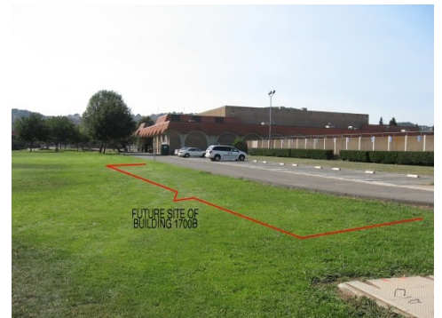
Prior to construction
